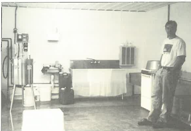
His milking parlor is small, about the size of a large stall within a modest barn. He milks two animals at a time in his 12' x 12' parlor. To construct the milking parlor, he converted a section inside a dirt-floored horse barn by pouring a concrete floor and applying pebble-textured dairy paneling to the walls. The milk room was formerly a tack room.
